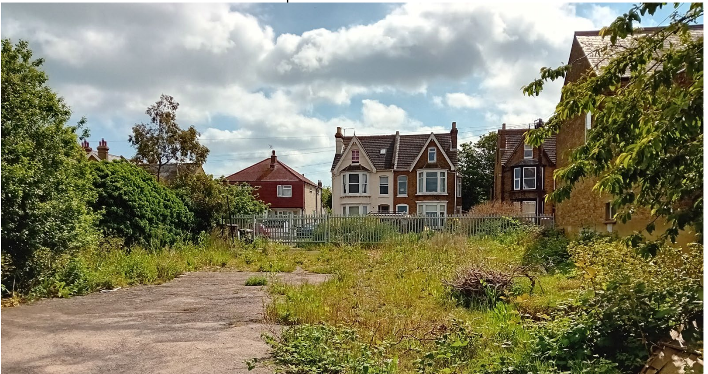
Below: Palisade fence erected on 17 th April 2023
